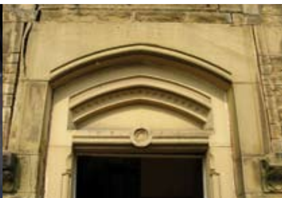
Elaborate carved stone door surround at Bridge Cottage, Lomeshaye Road, Nelson
