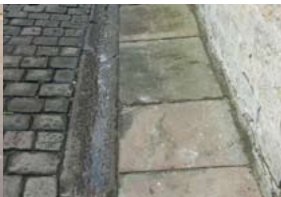
Stone paving and setts with a stone gully for drainage are typical of Pennine Lancashire
