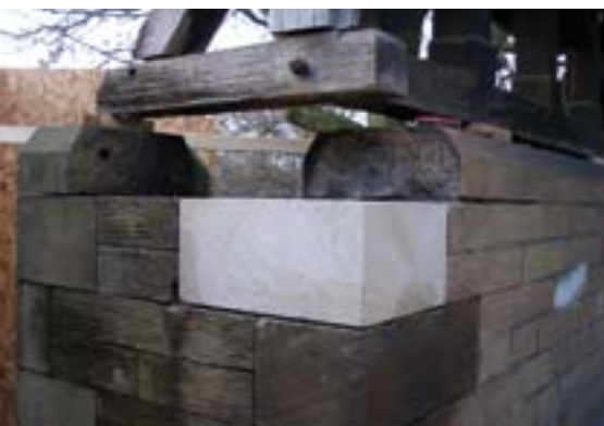
New dressed ashlar stone replace damaged stone
