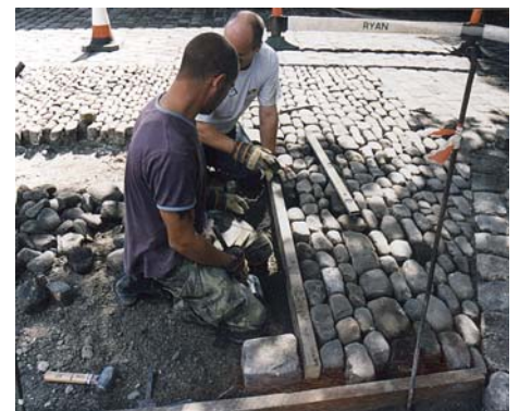
Restoring the cobbles in the farmyard at Park Hill.
