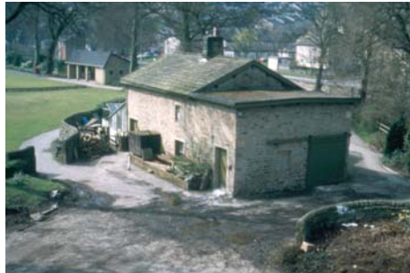
Views of Cottages before restoration. The pitched roof at one end has been replaced with a flat roof after a fire in the 1960s.
