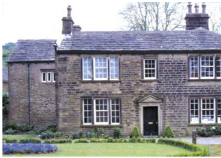
Known locally as the Clerk's Residence, the house became vacant in 1974, on the Reorganization of Local Government. It was leased to the Trust in 1977. The Trust restored the original glazing bars and took out the sham Victorian 'leaded' lights.
