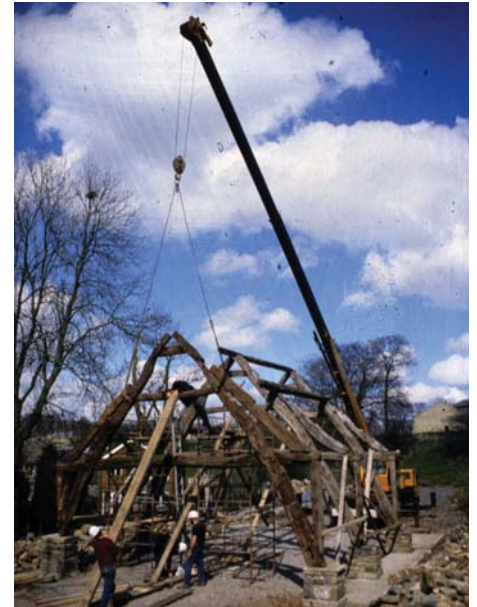
The huge frames being lifted into place with a crane.
