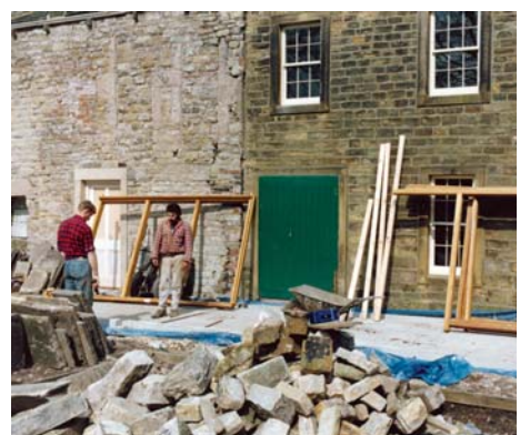
The construction of the Conservatory within the Walled Garden.
