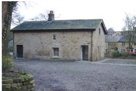
View of Cottages with pitched roof replaced in 1999.
