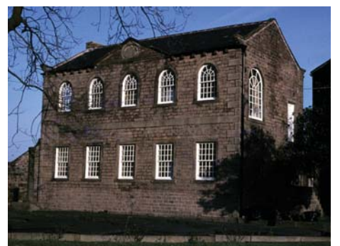
Old Colne Grammar School (built 1812) – one of the best in the county, was restored by the Trust and the Friends of Colne Heritage Centre between 1982 and 1984.
