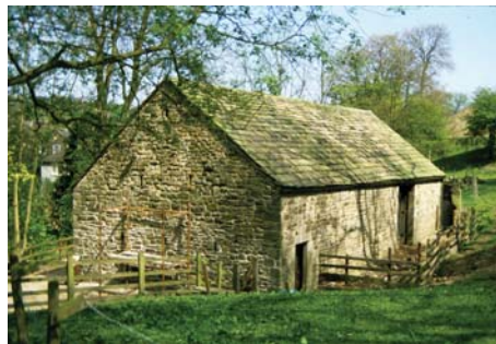
Originally the walls would have been constructed of timber with a roof of thatch but as it was considered a fire hazard to use these materials and also difficult to obtain ling thatch, it was agreed to build the walls in stone and roof it with stone slates.
