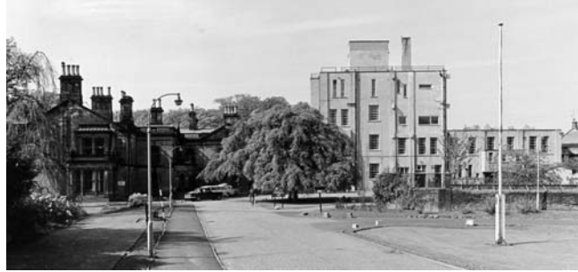
Reedyford Hospital was one of a number of buildings in the way of the M65 and had to be cleared.
