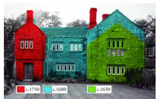
The front of Park Hill, showing the stages of construction
