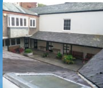
The courtyard of the Jacobean Hall. This is the oldest part and is in urgent need of repair to make it once more the hub of the Hall.
