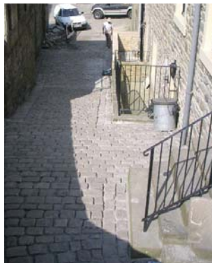
The reinstatement of cobbles and improvement work to cottages (before and after).
