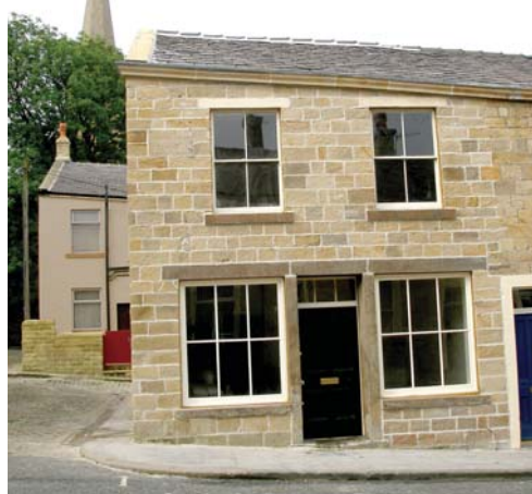
No. 2 Victoria St, before and after restoration.
