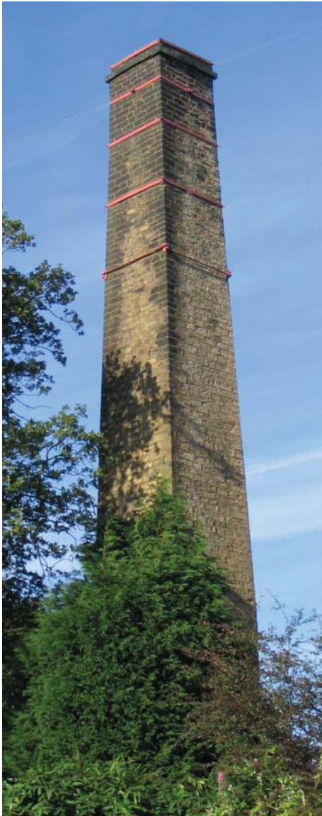
The square stone built Chimney at Higherford Mill is one of the earliest in Pendle, dated 1832. Later chimneys were built in brick and were usually round.
