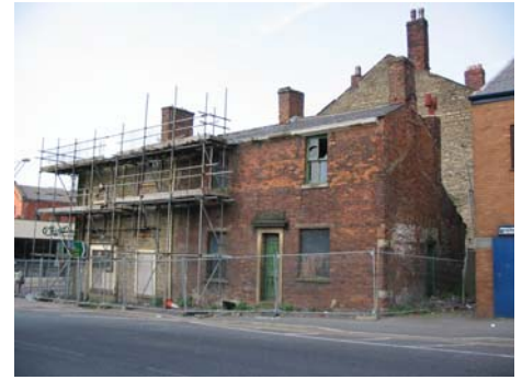
No. 3 Freckleton St. during restoration.
